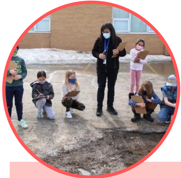
Grades 3/4 Erosion on school ground
